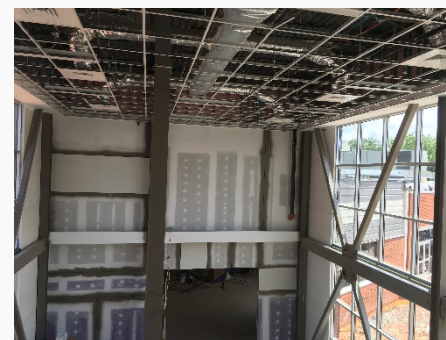
Lobby Window Wall, Duct, Ceiling Grid, & Prepped Gyp. Bd.
