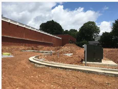
Curb and Gutter at Service Drive
