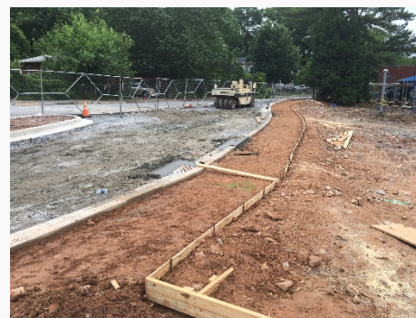
Prep. Framework for Sidewalk at Bus Loop
