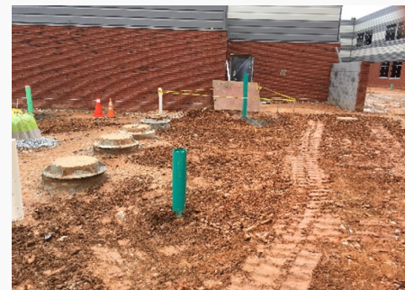
Manhole Covers to Finished Grade
