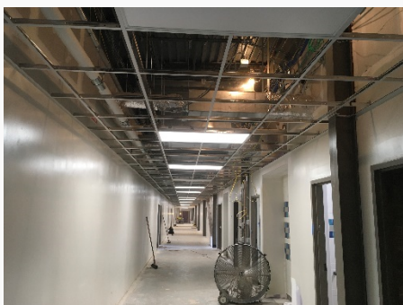
Ceiling Grid at New Building Upper Level
