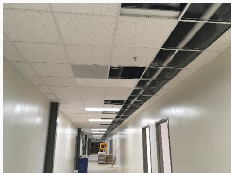
Ceiling Grid in of Upper Level Addition Corridor
